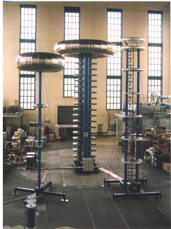
Fig. 4: Impulse Voltage Test System IP 360/3600 G (360 kJ, 3600 kV) with impulse voltage divider and chopping multiple spark gap, with a stage energy of 20 kJ being used for the LI test of power transformers up to 765 kV
