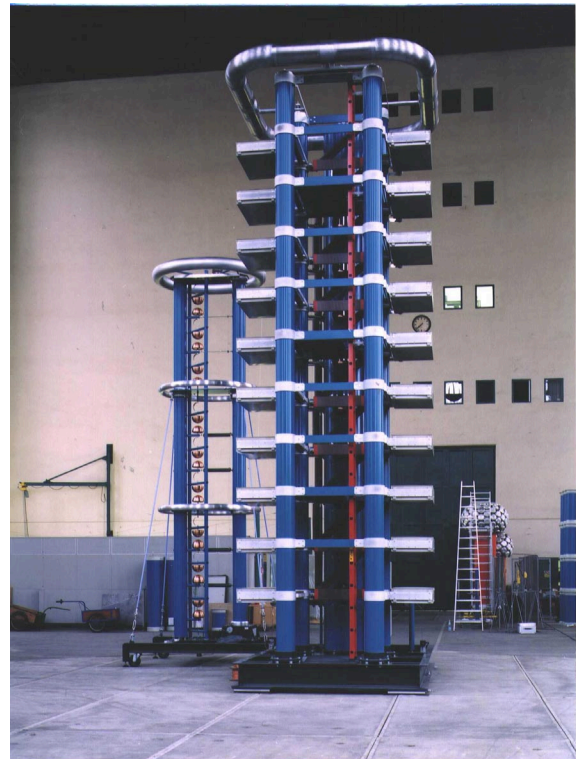
Fig. 5: Impulse Voltage Test System IP 150/2000 G (150 kJ, 2000 kV) with impulse voltage divider and chopping multiple spark gap, with a stage energy of 15 kJ being used for the LI test of power transformers up to 245 kV
