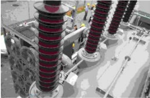
Figure 5: PD decoupling units of the monitoring system LDWD-6 installed on a power transformer
