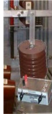
Figure 6: PD couplers installed in the bushar of a high voltage generator
