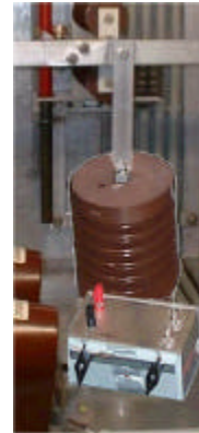
Figure 6: PD couplers installed in the busbar of a high voltage generator
